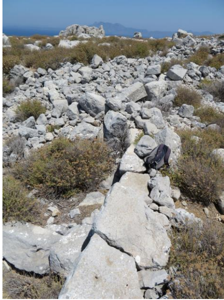
Looking along the wall from A to B
