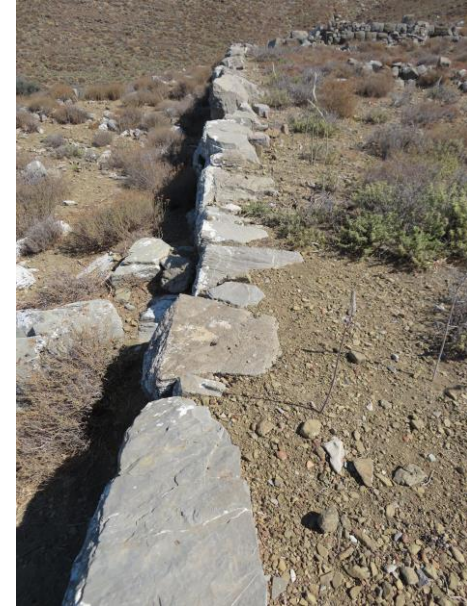
On top of the seaward wall looking from B to C
