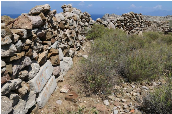
Perimeter walls of the enclosure are random stone
